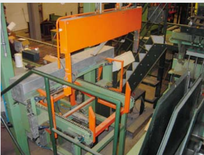
A convex mirror has been fitted so that an operator can see what is happening on the lower level (A.S.).
